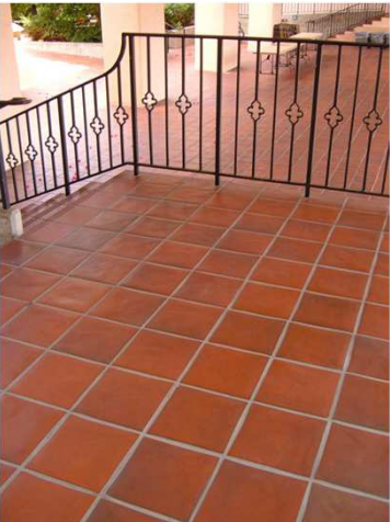
Quarry Tile - Main Aisles and Vestibule
